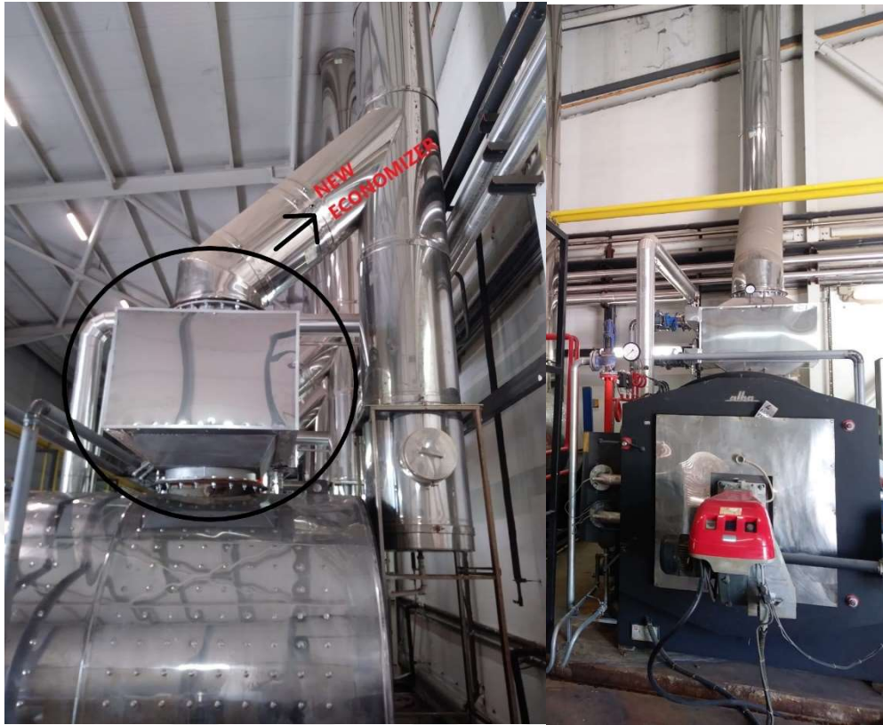
Figure 4.2. Photo of the installation of new economizer.
