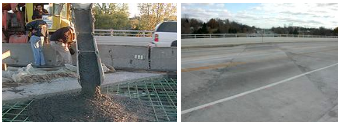
(a) during construction
