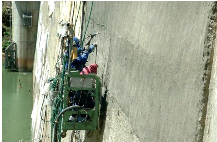
Figure 2.15 Spray repair of the Mitaka Dam with ECC for water-proofing (Sakata et al., 2004)
