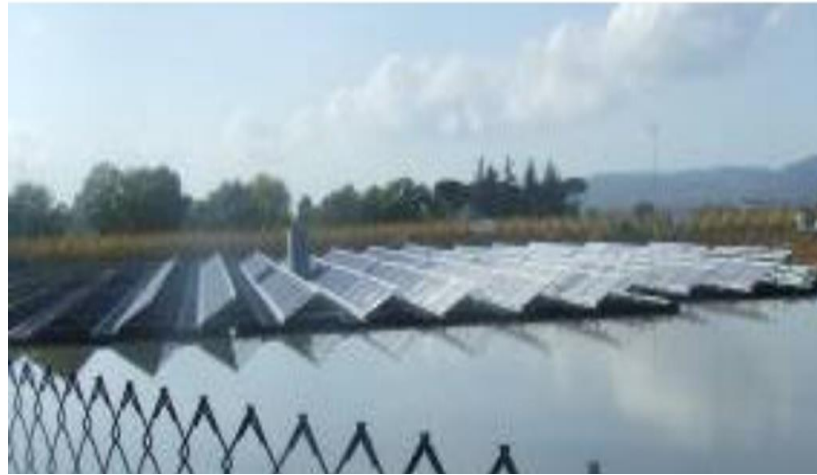
Figure 4.20 First solution system which is built in Suvereto, Italy (Cazzaniga et al. 2012)
