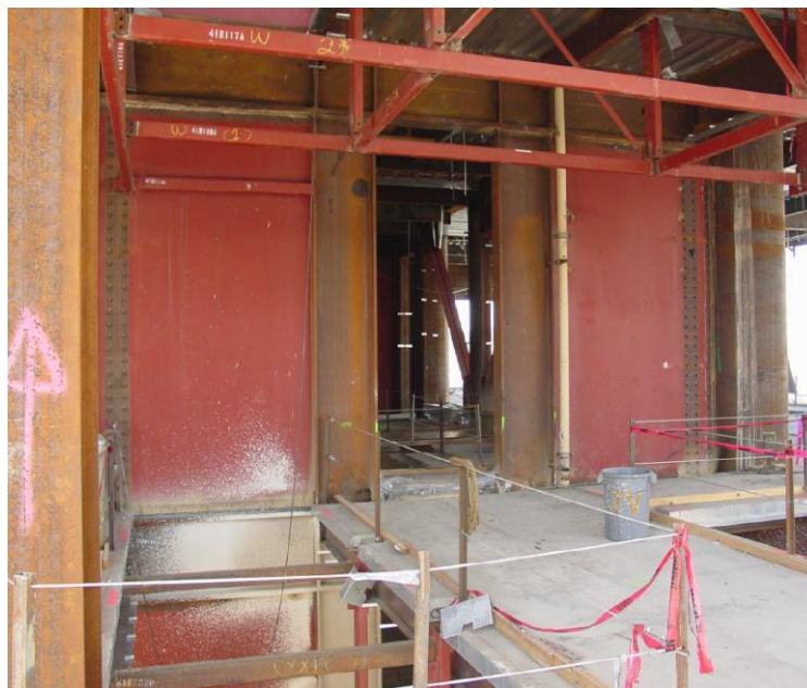
Figure 1.2 Steel plate shear wall element (Stankevicius, 2011)
