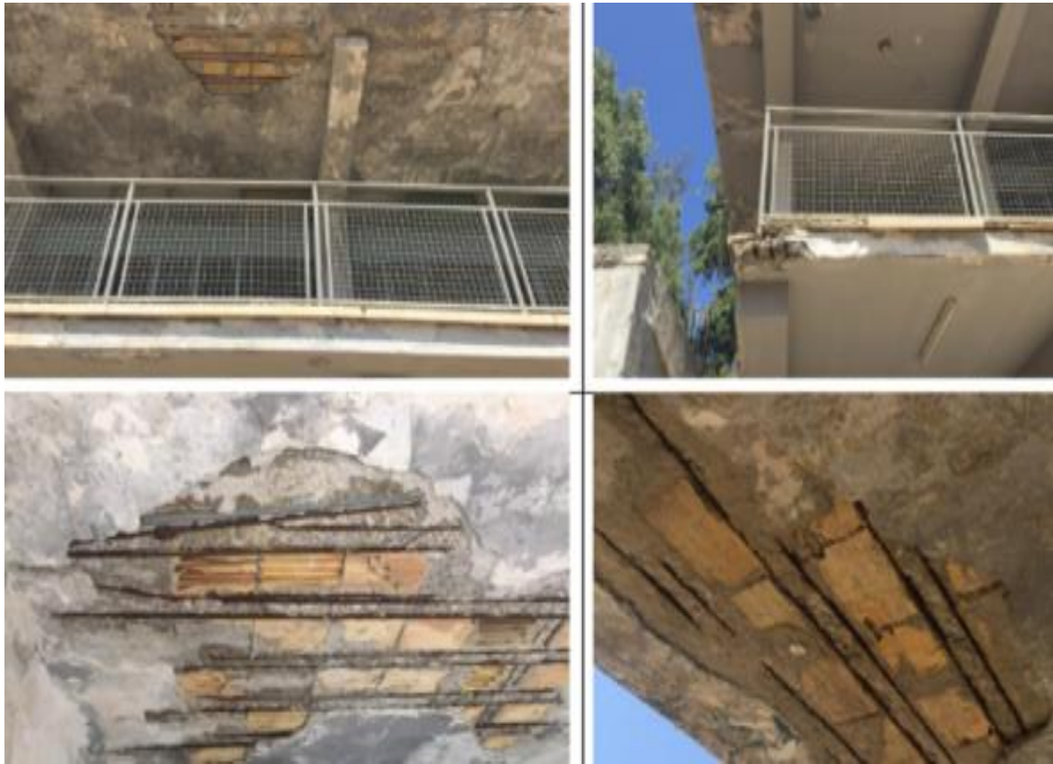
Figure 2.1: RC slabs without bond strength (Lefke high school).
