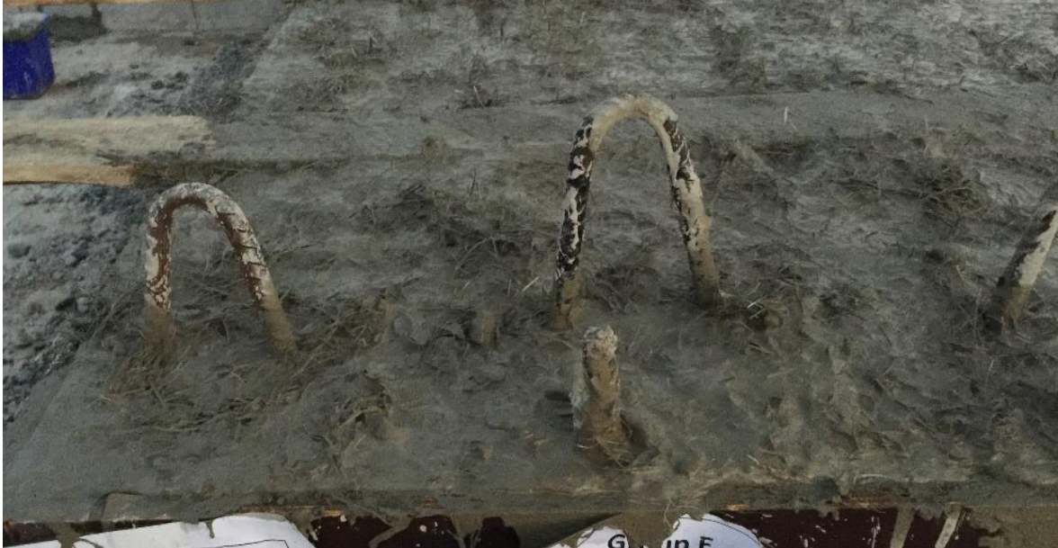
Figure 3. 14: Poured concrete with fibers.
