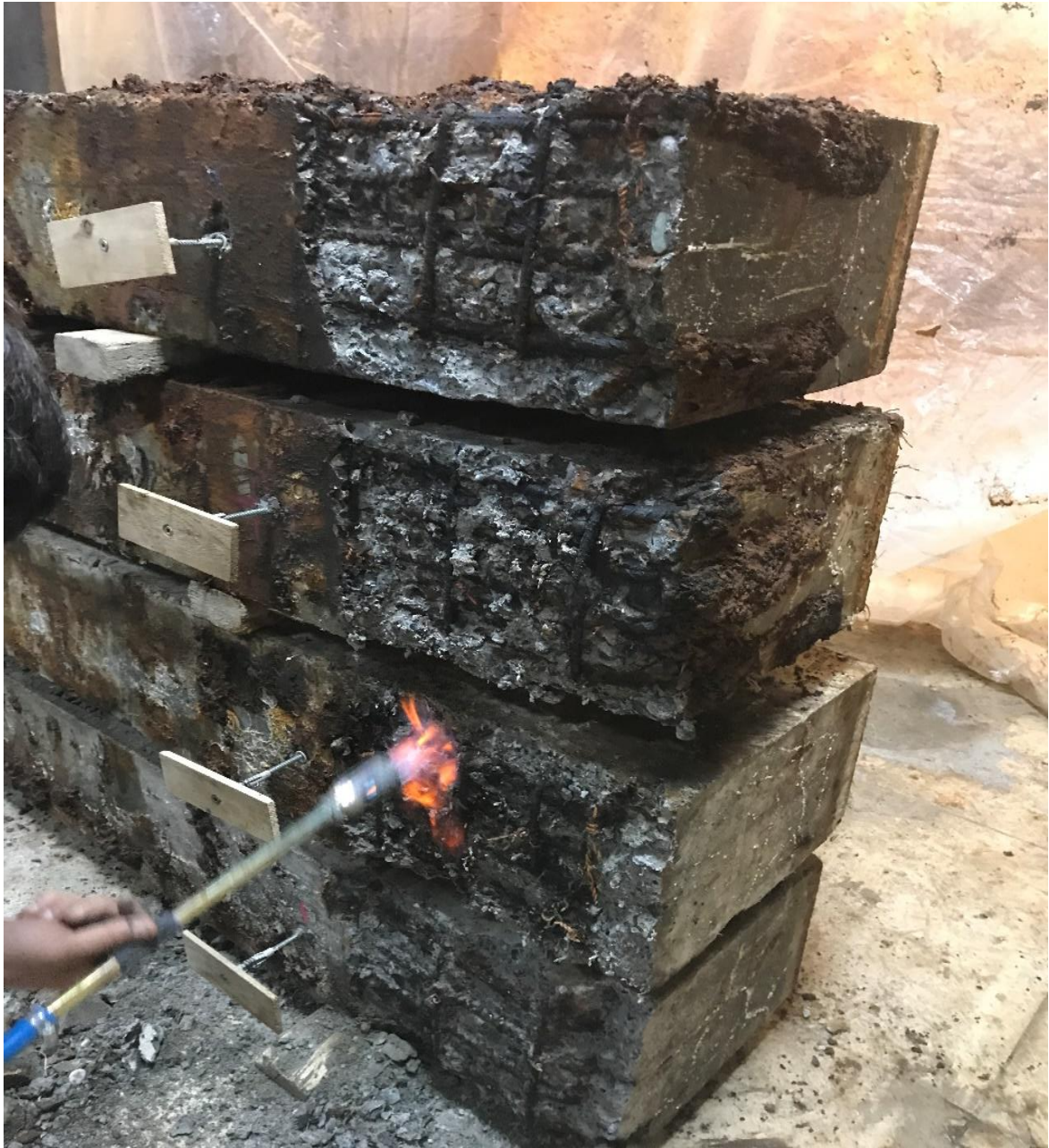
Figure 3. 21: Cleaning and repairing of support.
