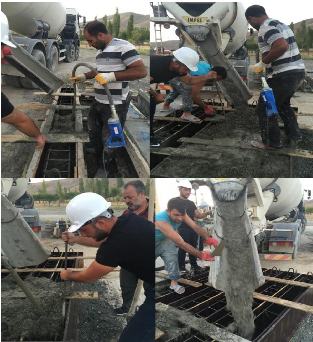
Figure 3. 12: Pouring and vibrating concrete process.
