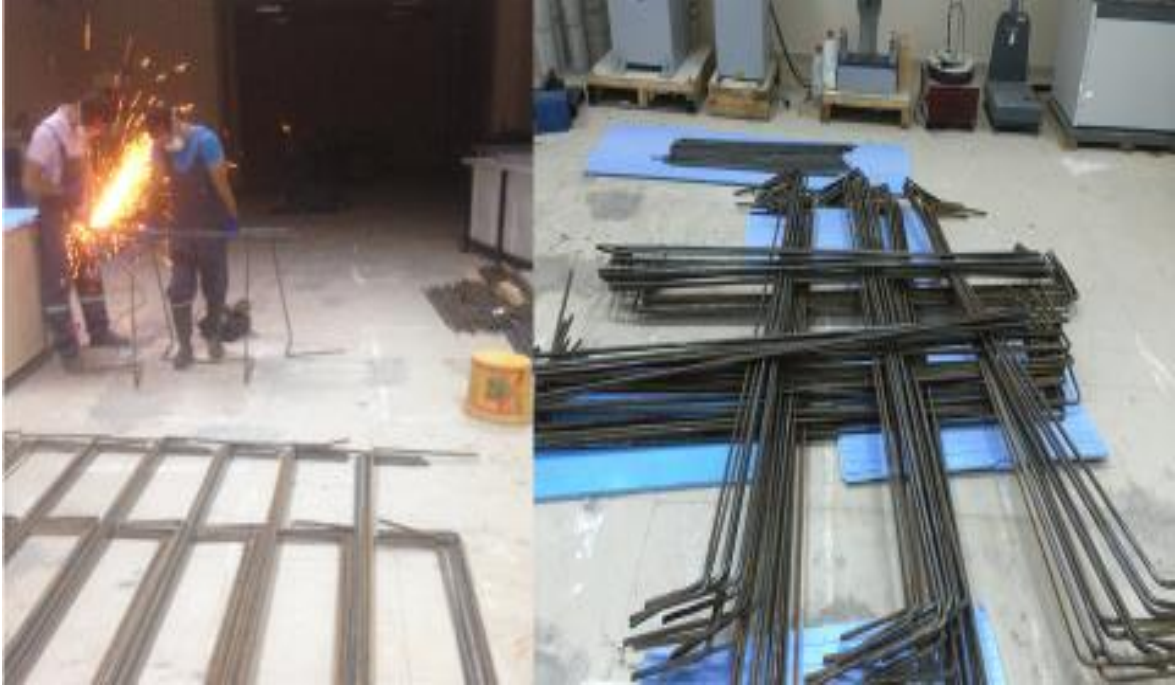
Figure 3. 4: Cleaning phase of reinforcement.
