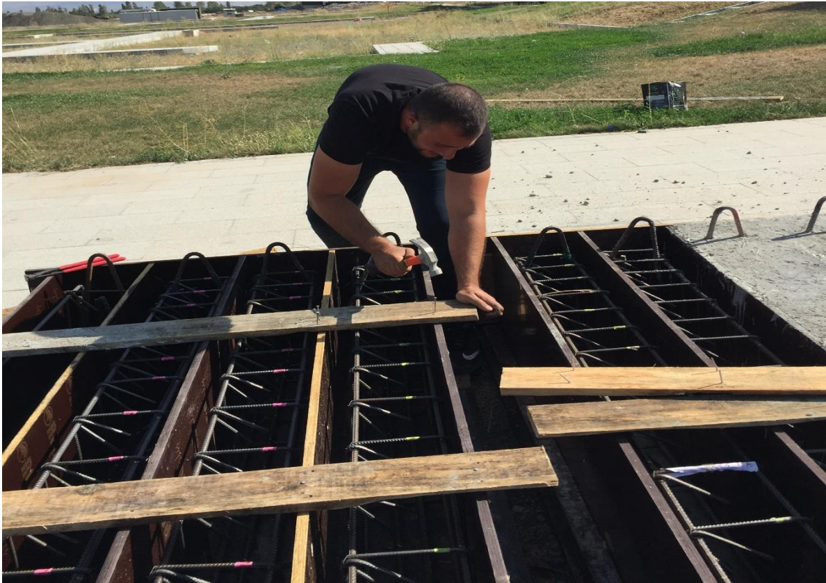
Figure 3. 3: Strengthening of moulds.
