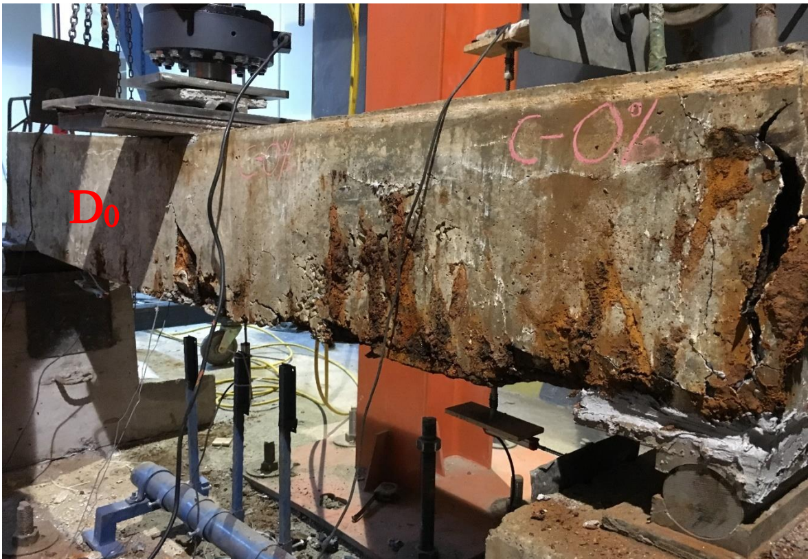
Figure 11. Load-displacement relationships of corroded RC beams for D0
