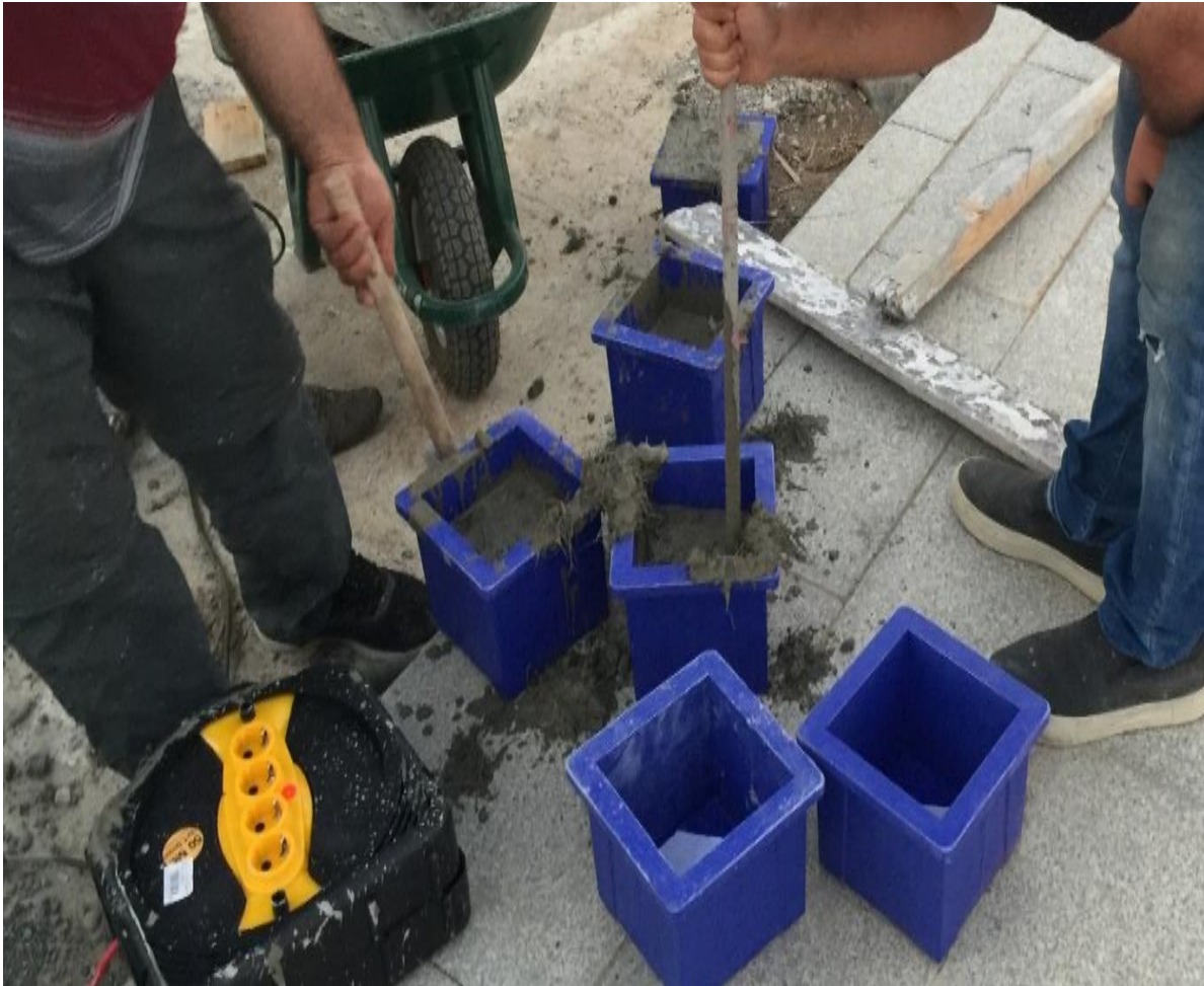
Figure 3. 13: Compacting the concrete in the cube moulds.
