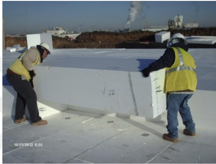
Figure 2.10. Placement process of EPS geofoam (Puppala et al., 2019)
