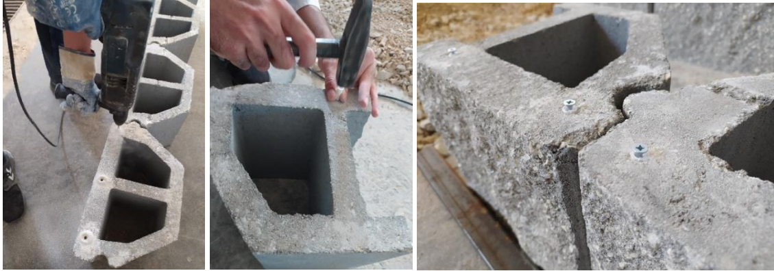
Figure 8.3. a) Drilling with a drill, b) Embedding anchors, and c) Placing screws in modular blocks
