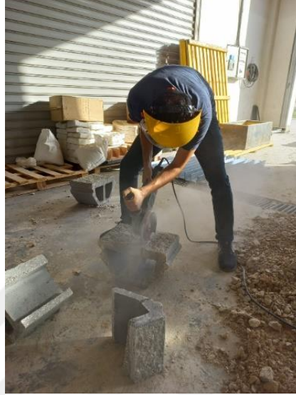
Figure 8.2. Cutting process of modular block
