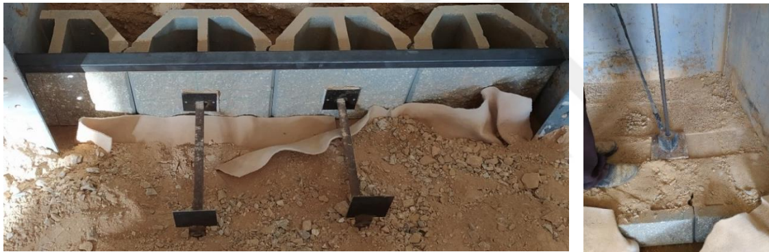
Figure 8.9. a) Placement of modular blocks, and b) Compaction process with a compaction hammer.
