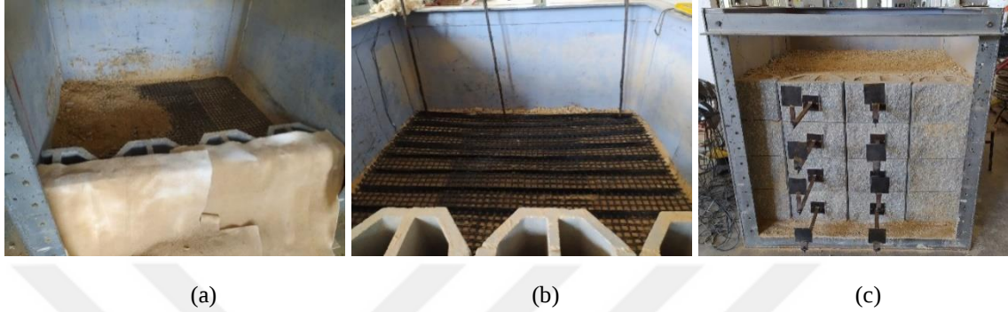
Figure 8.10. a) Filling process of the backfill material, b) Tensioning of the sample with the help of steel rods, and c) Constructed MSE wall
