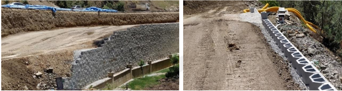
Figure 5.1. The construction site of the MSE wall
