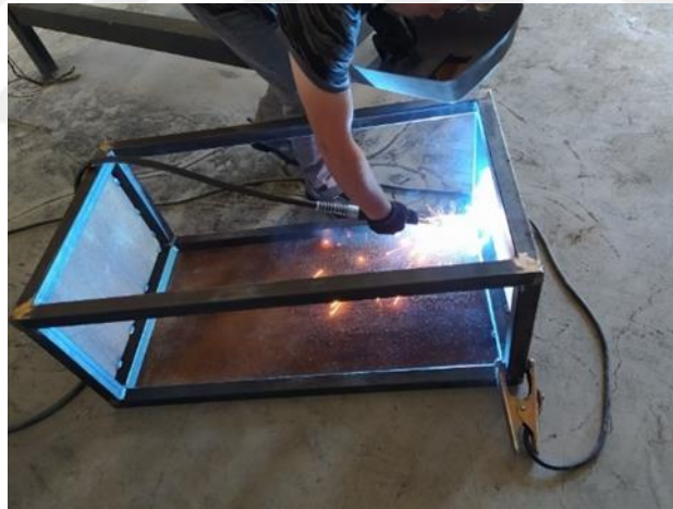
Figure 6.1. Welding of metal plates
