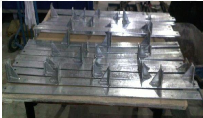
Figure 4.7. Steel strips with anchoring elements (Esfandiari & Selamat, 2012)
