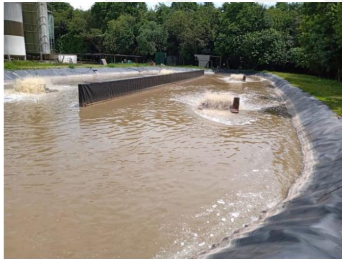
Figure 2.8. HDPE geomembrane used in sewage pond (Lavoie et al., 2020)
