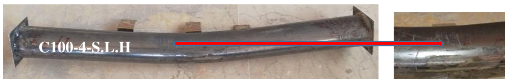
(C) Sample no three C100-4-SLH of the third group failure modes
