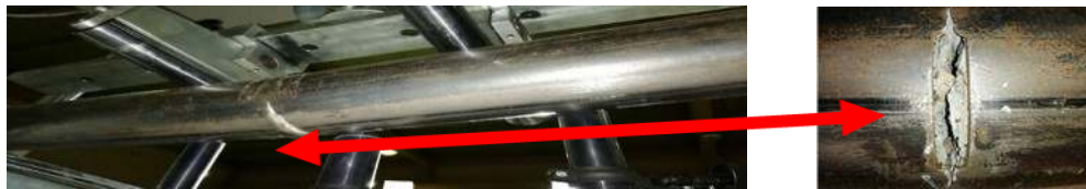
(D) Sample no four C100-4-BLV of the first group failure modes
