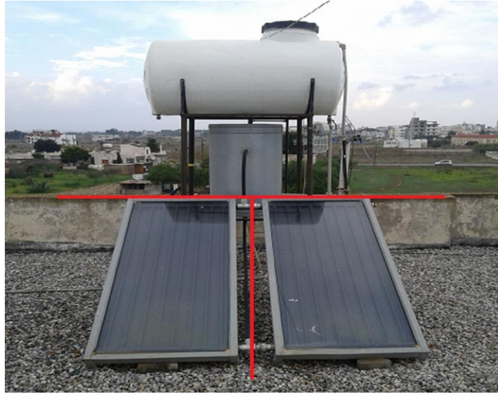
Figure 38. The Azimuth Angle of Collectors in Haci Ali Apartment
