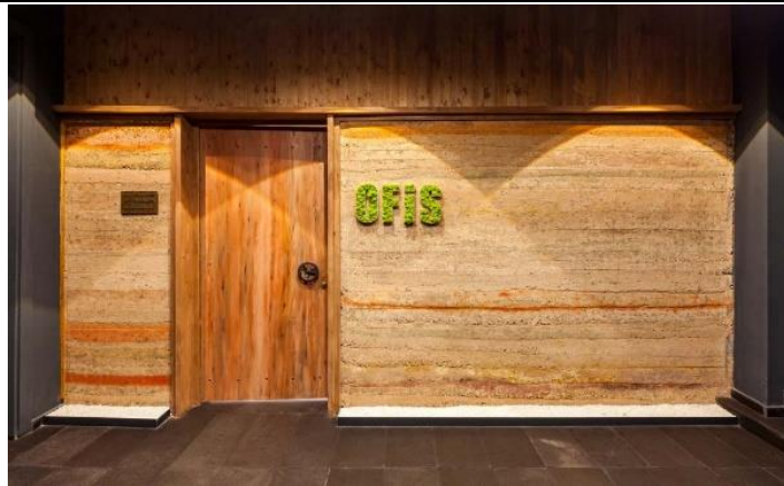
Figure 3.11: Alker Wall in BKM. Photograph by Sahir Uğur Eren.
