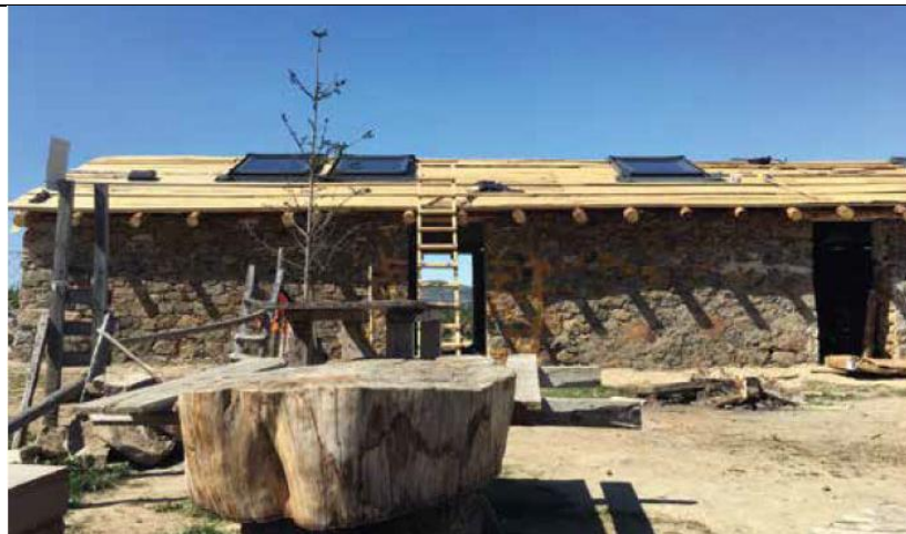
Figure 3.10: A photograph from Yayla House Construction Site
