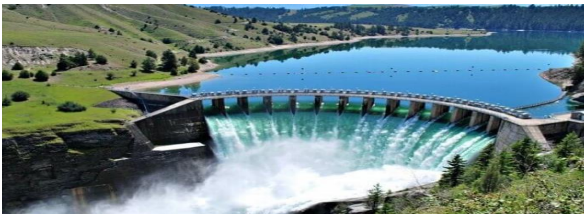
Figure 1.7. Hydroelectric power plants
