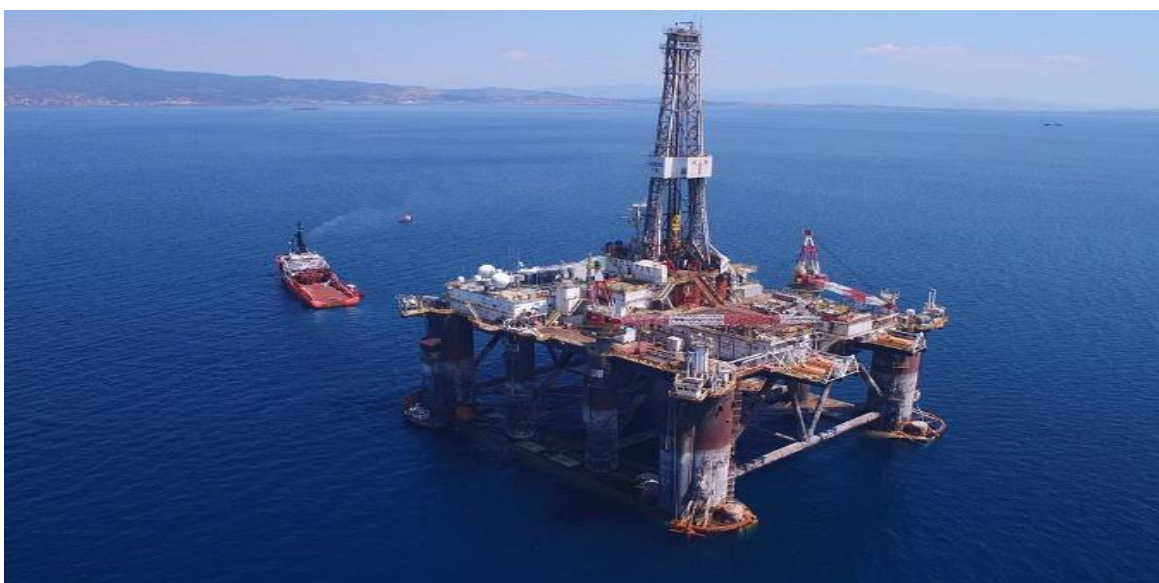
Figure 1.3. Natural gas station
