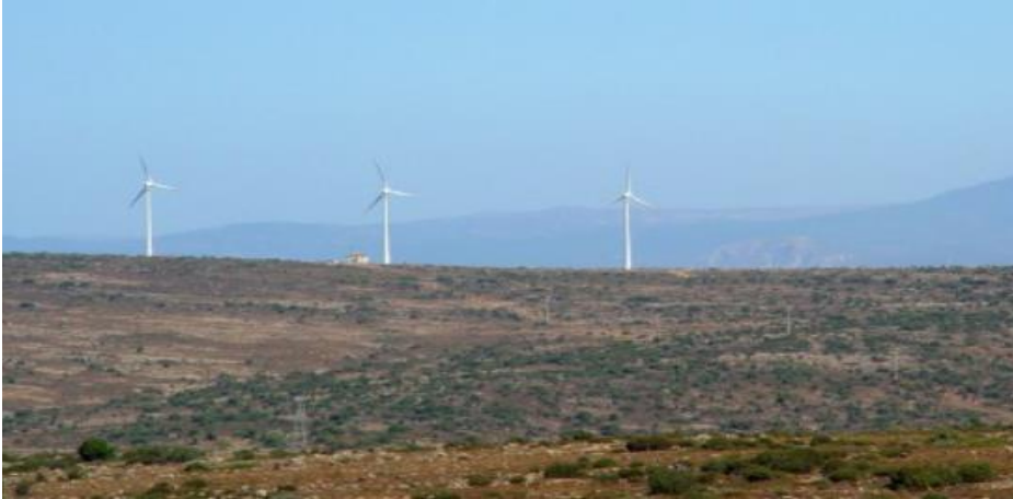
Figure 1.12. Alize-Çeşme wind power plant
