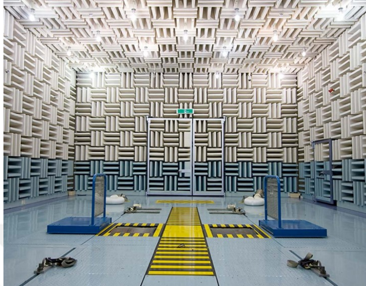
Figure 2.2: Semi Anechoic Room.
