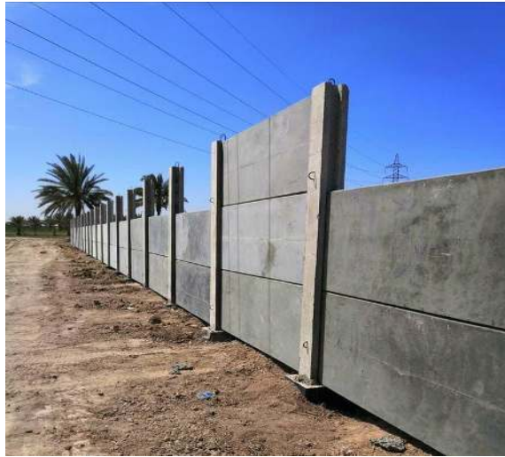
Figure 2. Example of production of precast in Iraq.
