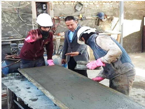
Figure 43. Putting the concrete mixtures in a specific mold to form precast.
