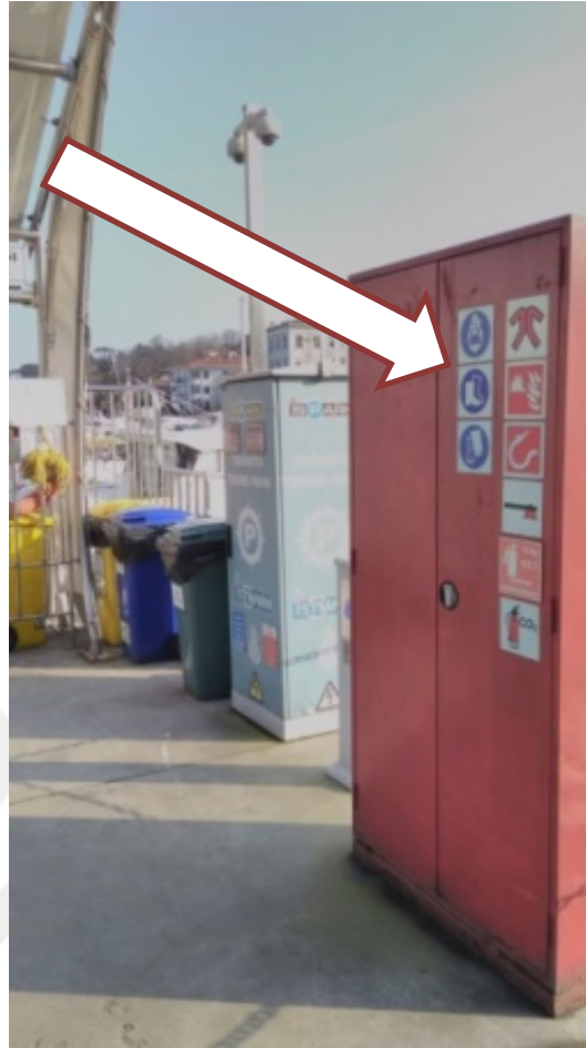
Figure 19: Accessible Maintenance and Safety Equipment in İSTMARİN Tarabya Boat Park
