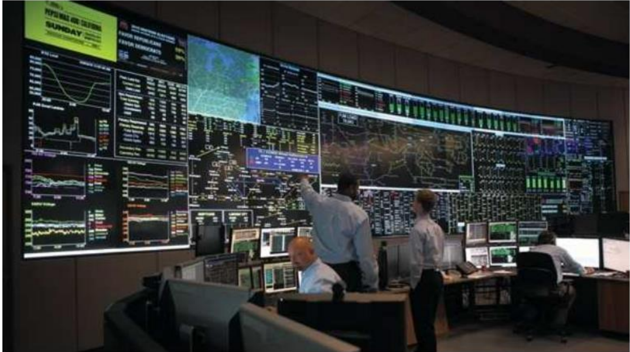
Figure 3.1: Smart grid control centers [4]
