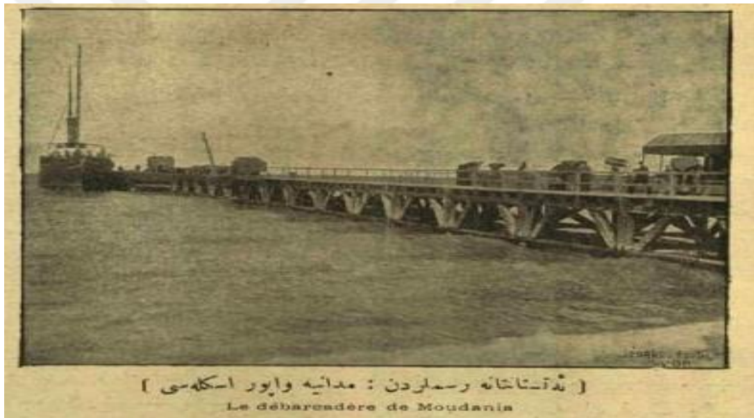
Figure 15. Pier of Mudanya, Servet-i Fünun 291 (1896), 177.
