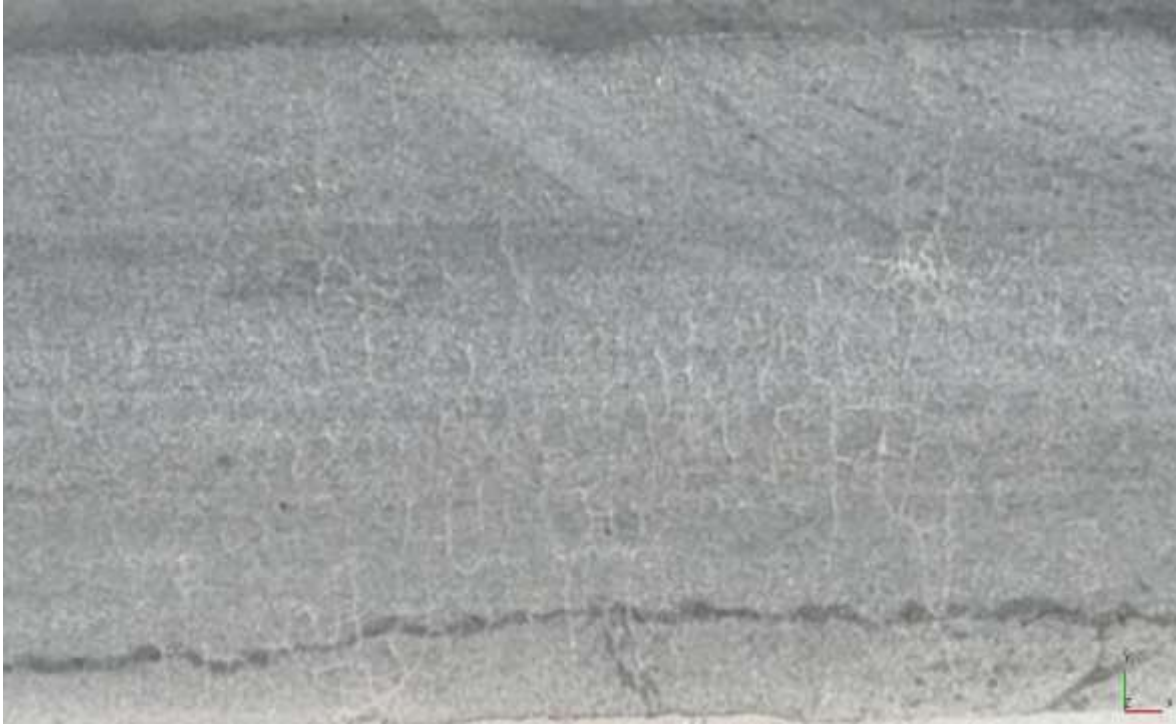
Figure 4.4: The Cracked and Uncracked Areas Before the Crack Mapping Process.
