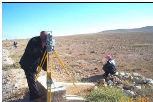
Photo 3. Use of Total Station Maintained the Accuracy in Layout of the Structures
