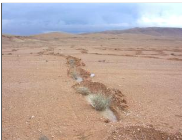
Photo 16. Runoff at the Shrub Location Satisfies that the MCWH Functions Properly
