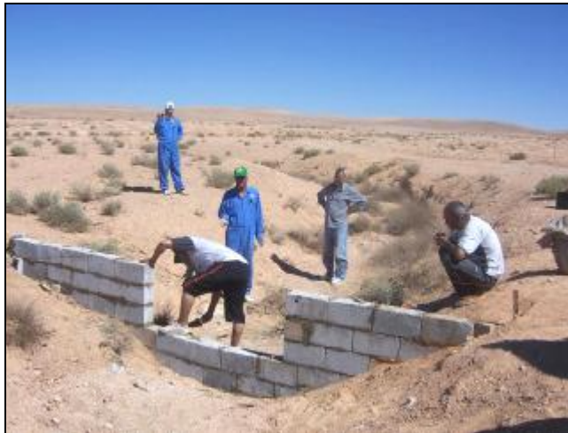
Photo 5. Construction of Weirs in Gullies and Automatic Data Loggers Facilitated Real-time Measurement of Stage Hydrographs
