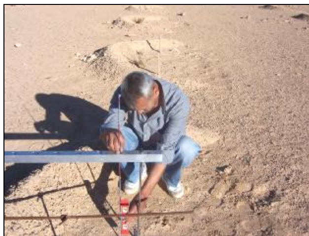
Photo 15. Precision in Measurement Requires Check for Horizontal and Vertical Controls for Ridge Bridge Frame
