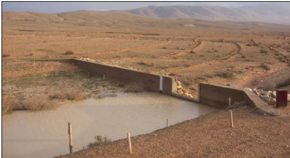
Figure 3.14. Sharp-crested Weir and Automatic Data Sensor to Record Real-time Stage Hydrograph.
