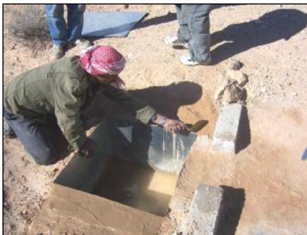
Photo 11. Installation of Runoff and Sediment Tanks in Progress
