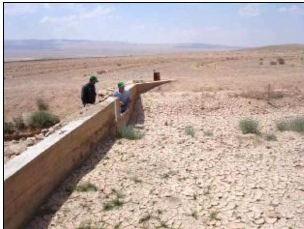
Photo 8. Sediment in Front of the Weirs was Measured for each Runoff Event
