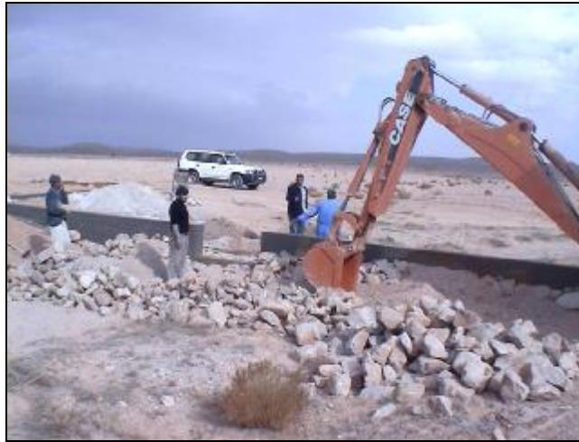
Photo 4. The Work on the Construction of Weir is in Progress
