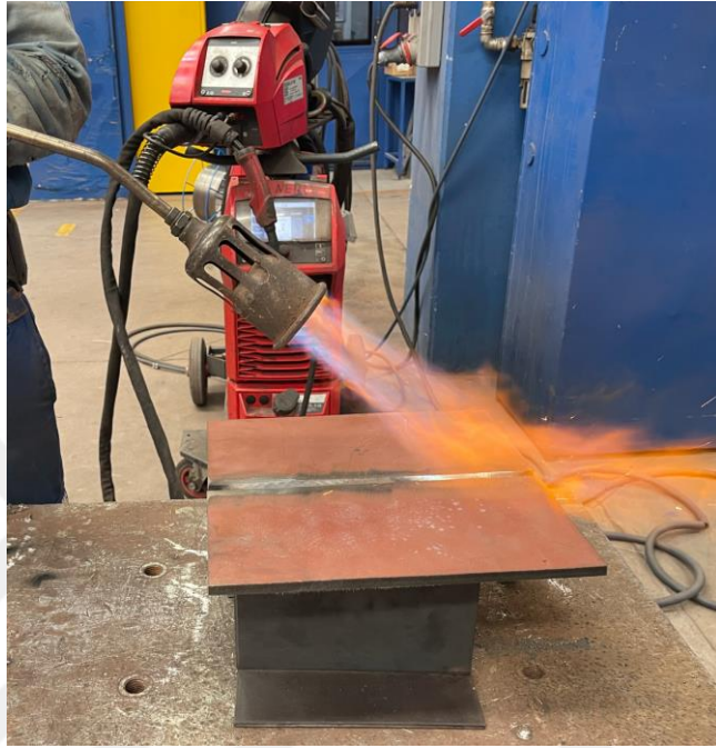
Figure 3.2. Preheating With Propane Torch
