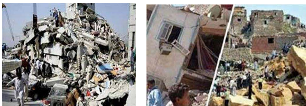
Figure 2.2 Damages of Egypt earthquake , 1992
