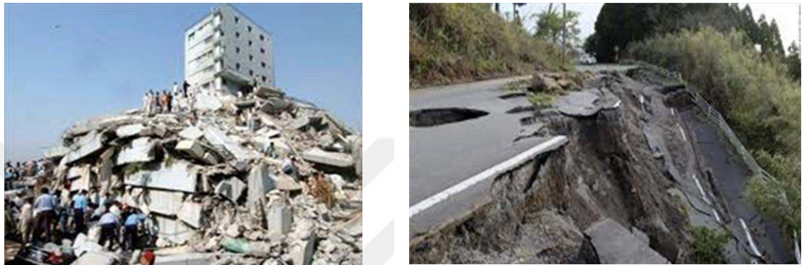
Figure 2.3 Damages of Lebanon earthquake
