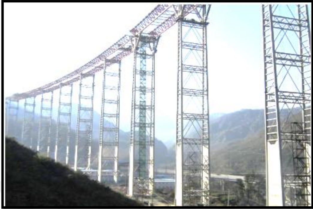
Figure 2.16 Built- up columns used for continuous beam bridge (Ganhaizi Bridge, China) (Huang, 2015)
