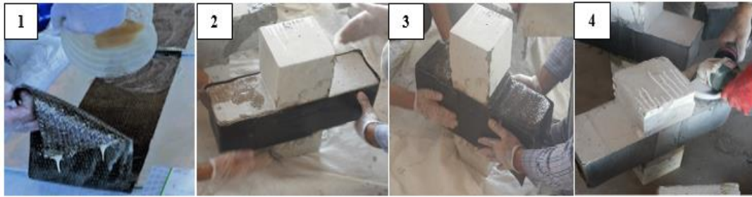
Figure 4.4 Configuration steps of bonding surface and applying the BFF with epoxy
