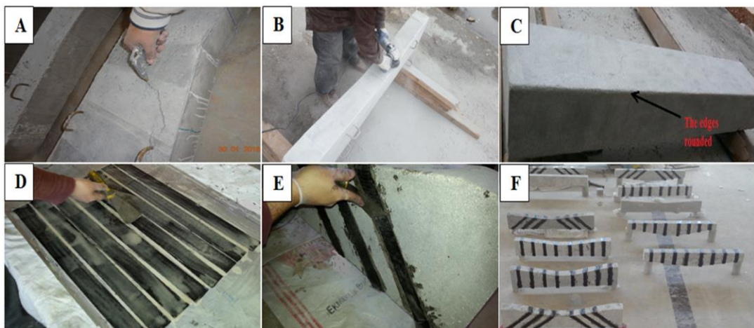
Figure 3.12 Photos show some steps of rehabilitation and strengthening
