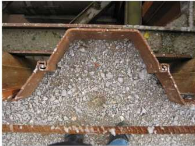
Figure 2.14. Steel sheet-pile wall [9]
