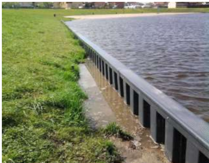
Figure 2.15. Vinyl sheet-pile wall [9]
