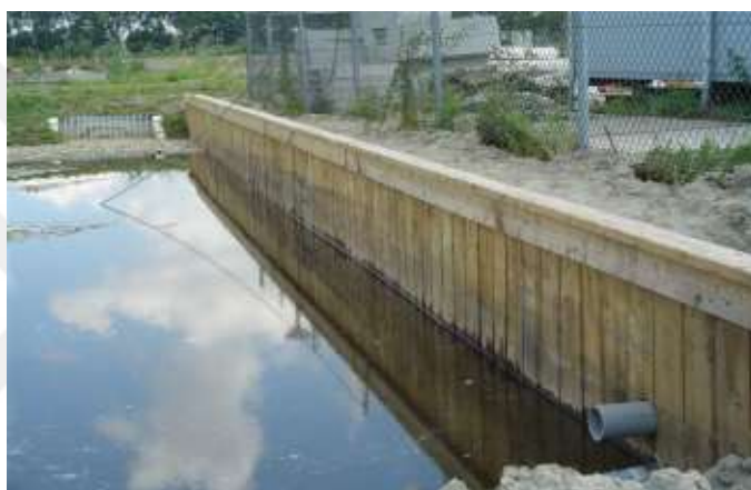
Figure 2.11. Wooden sheet-pile wall [9]
