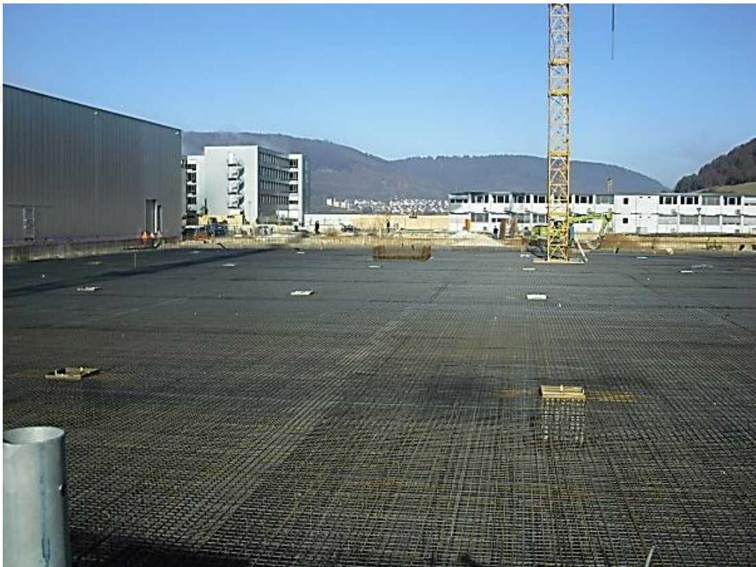
Figure 2.8 The raft foundation for 30 m building (Structurae, 2017)
