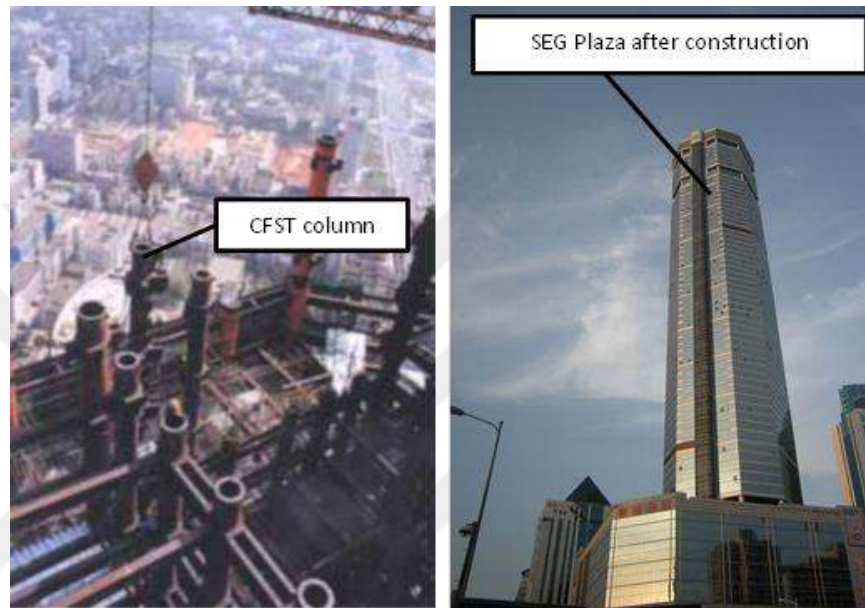
Figure 2.32 SEG Plaza constructed with CFST column (Wang, 2014)
