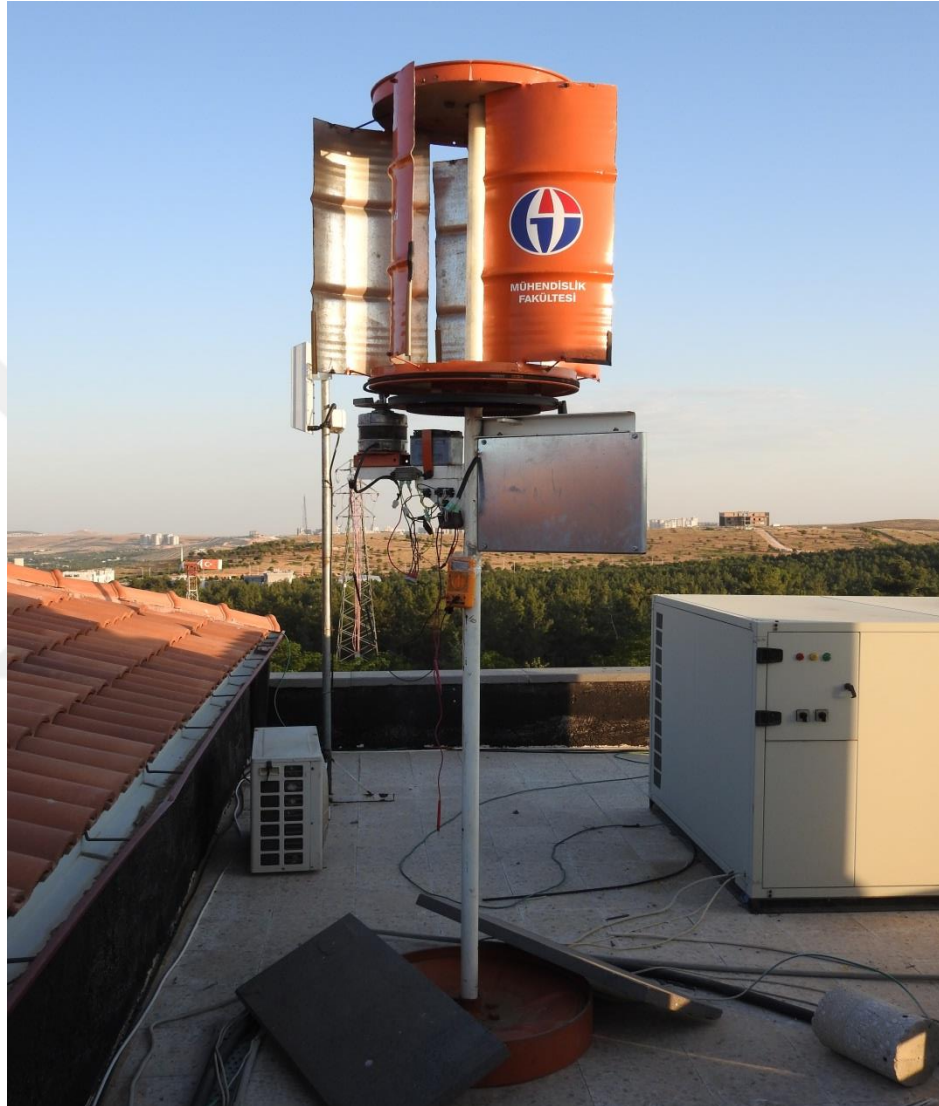
Figure 3.1 The model one of turbine Savonius.
