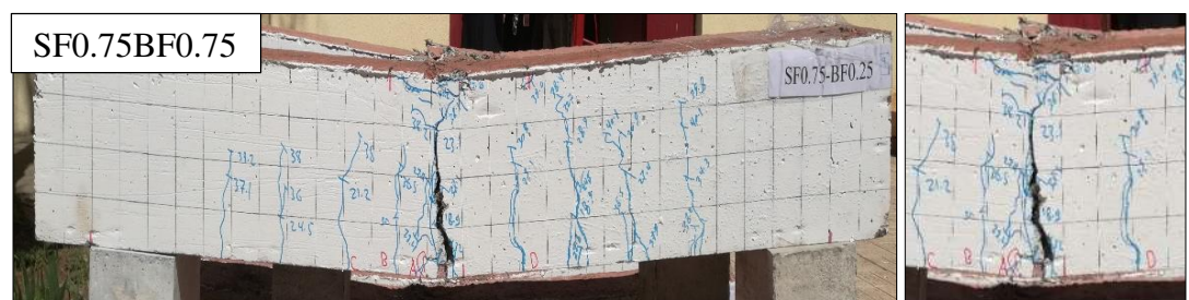
(c) Crack pattern and failure mode for group B
