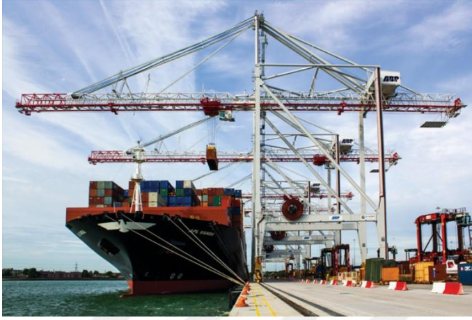
Gantry Vinci (STS)
