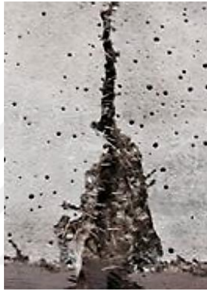
Figure 4.17. Failure state in MSF reinforced UHPC after fracture energy test
