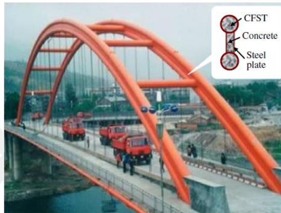
Figure 2.32. Wangcang East River Bridge in China [42]
