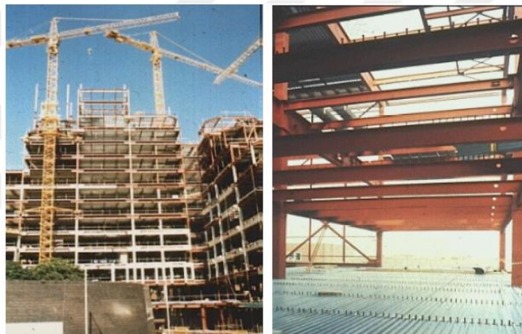
Figure 2.29. Composite multi-storey steel-framed constructions (Building used for commercial located in London and car industry factory building in Germany) [137]
