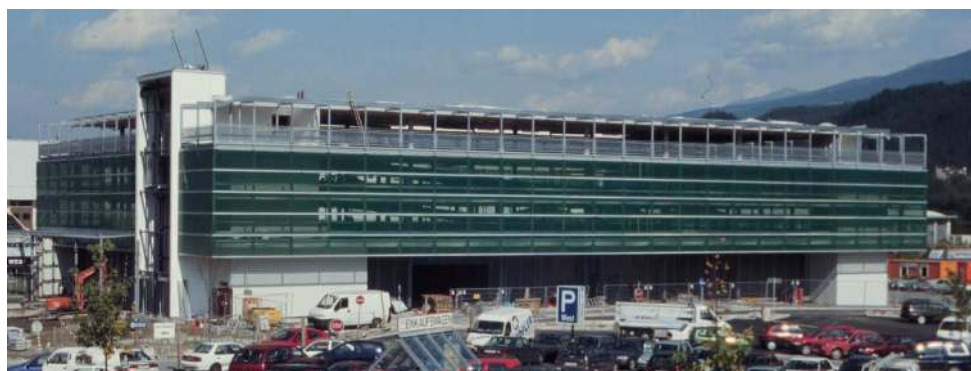
Figure 2.27. Parking deck “DEZ” in Innsbruck – Austria [136]
