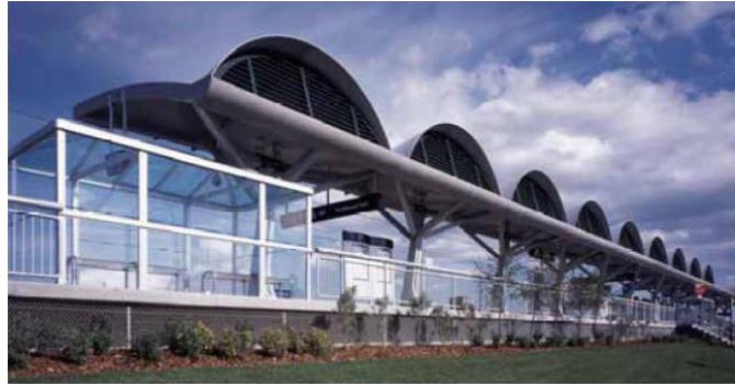
Figure 2.18. Shawnessy LRT station with UHPC canopies [97]
