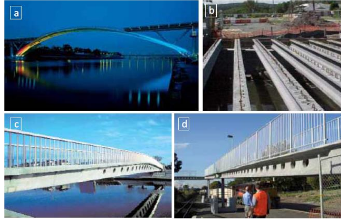
Figure 2.17. Examples of UHPC bridges and footbridges: a) Footbridge of Peace in South Korea, b) Shepherd Creek Road Bridge in Australia, c) Sakata Mirai footbridge in Japan, and d) Papatoetoe footbridge in New Zealand [97, 103, 110]
