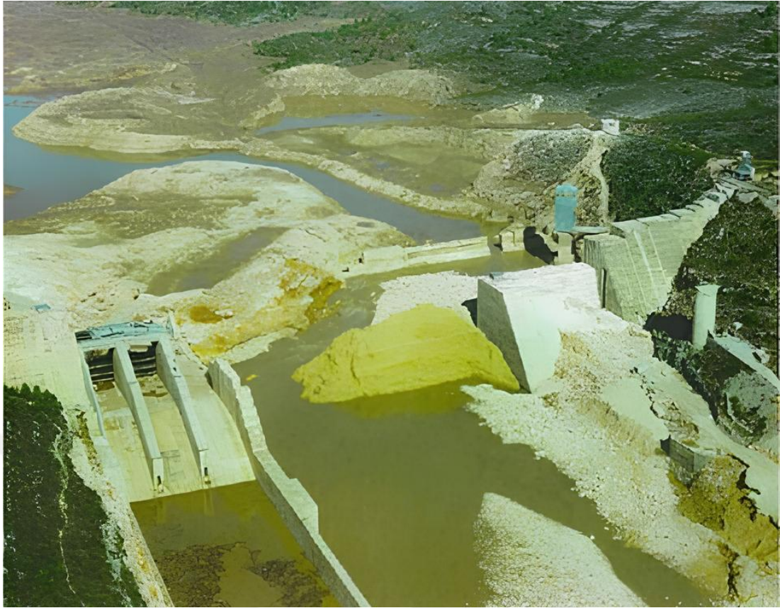
Figure 2.4 Breaching of the Tous Dam (Talukdar and Dey, 2019)
