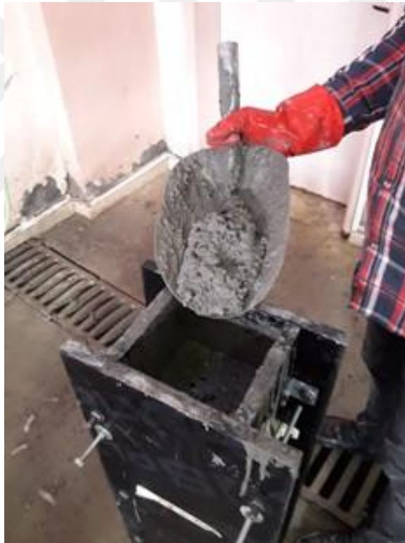
Figure 3.4 The specimens during casting
