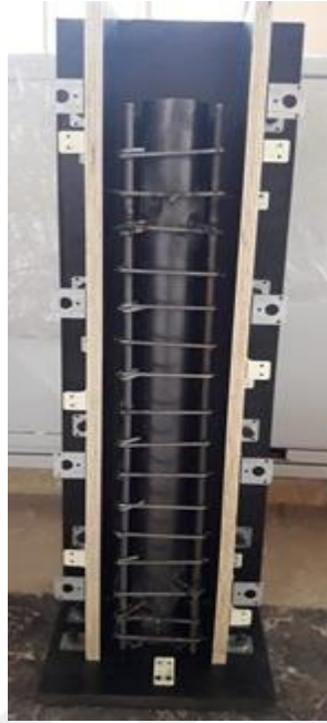
Figure 3.5 The specimen before casting (front view).
