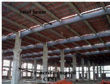
Figure 1.1 Concrete-encased CFST column with steel beams
