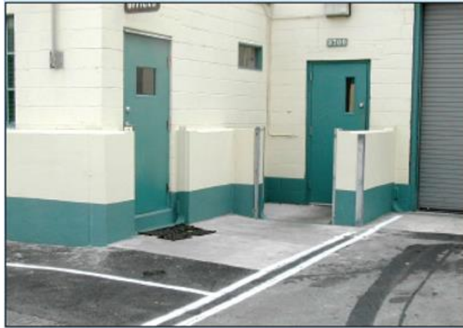
Figure 4-6 Adding an extra layer wall around the house's external wall [62]
