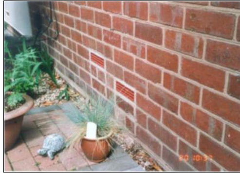
Figure 4-11 An example of air brick [60]
