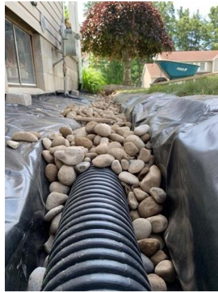
Figure 4-4 External drainage system [63]
