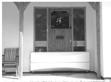
Figure 4-10 Using a temporary door protection barrier [60].
