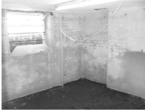
Figure 4-2 Basement tanking [60].
