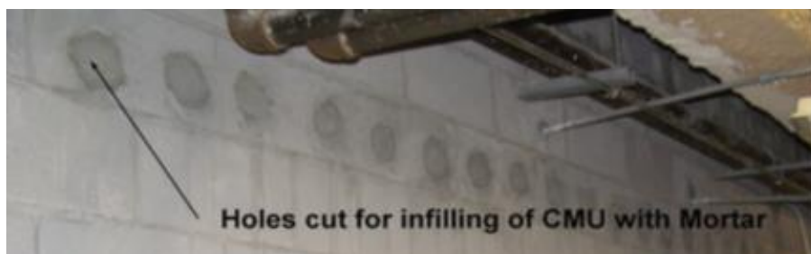
Figure 4-7 An example of a grouted masonry wall [62].
