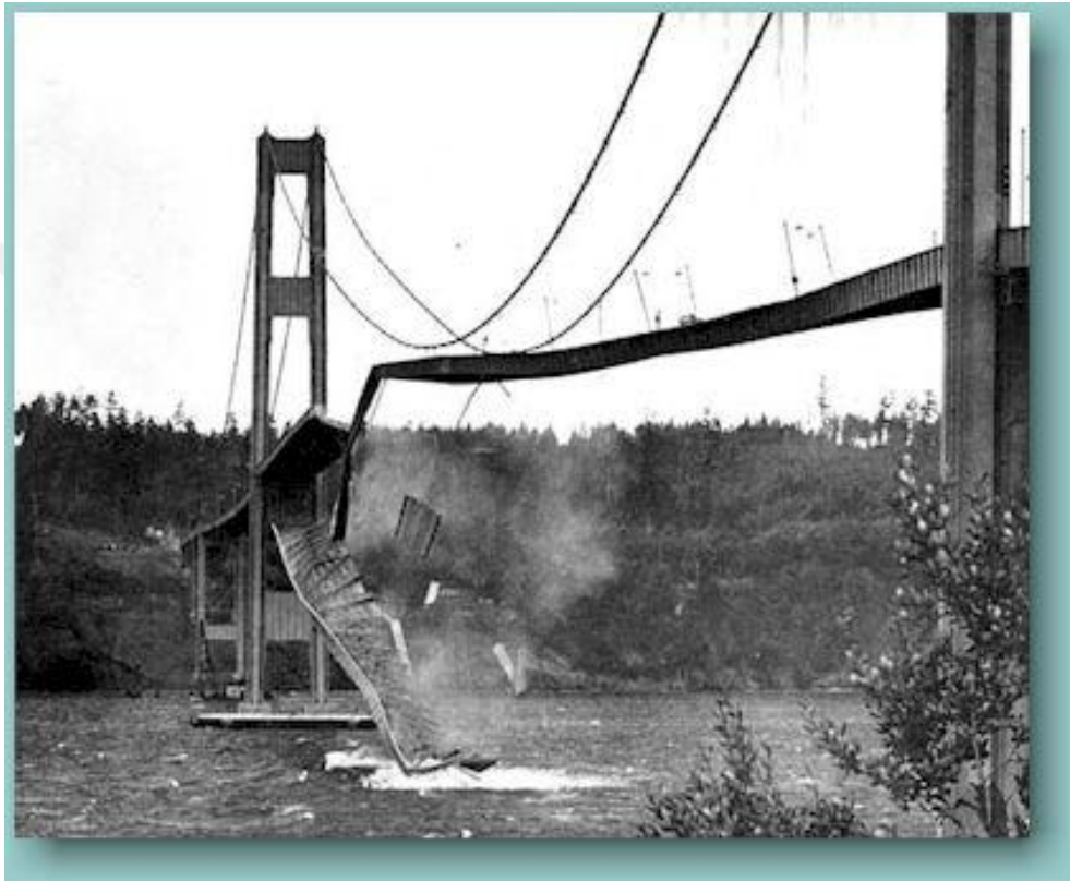
Figure 1.4. The collapse of Tacoma Narrows Bridge because of vortex lock-in ( http://www.lib.washington.edu/specialcollections/collections/exhibits/tnb )
