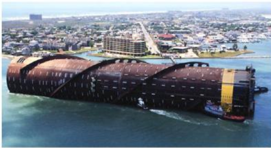
Figure 1.5. A spar with helical strakes ( http://www3.imperial.ac.uk/vortexflows/research/fluidstruct/vivofrigidstructures ).
