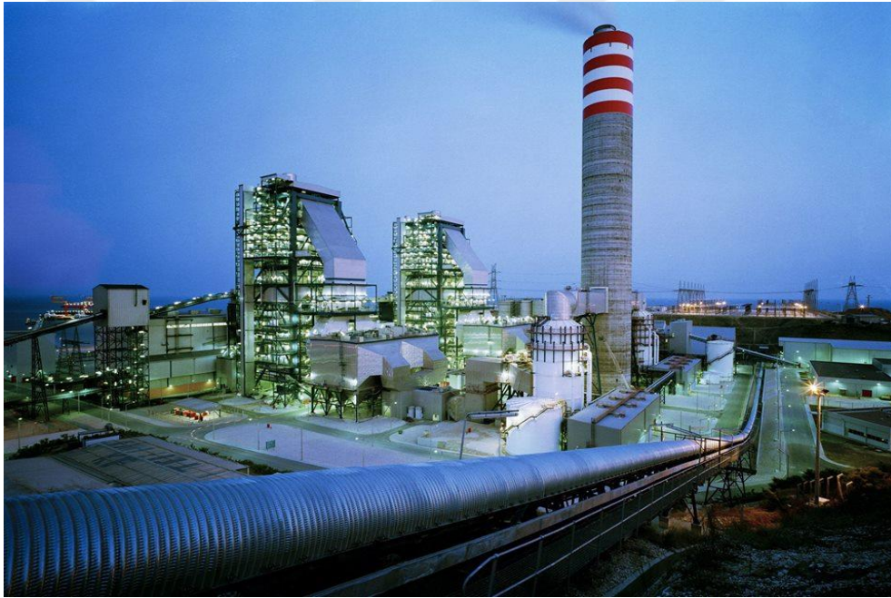
Figure 3.2. Coal fired steam power plant
