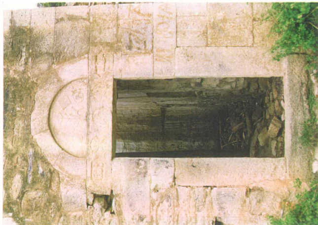
FIGURE.2.47. The Door of the Tower House
