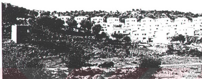
FIGURE.3.11. The improper built-up near the Tower House 51 in Sazlıca
