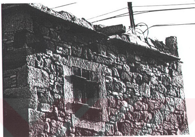
FIGURE 2.143. Decorative Roof Corners, Flatstone Eave, Rain Gutter
