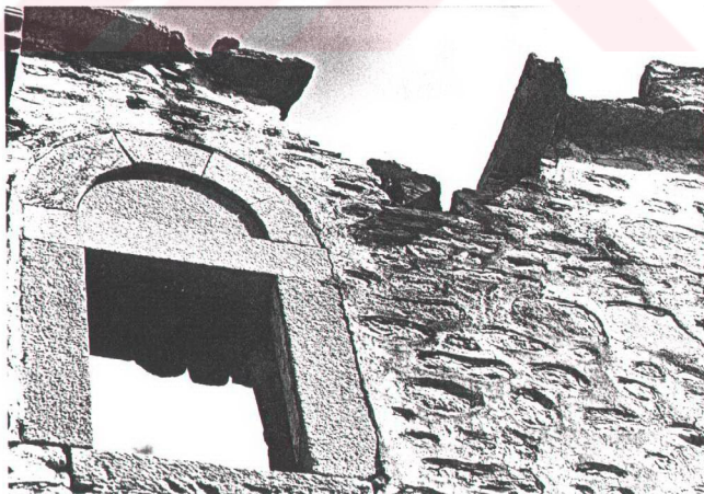
FIGURE.2.132. Flatstone Eave, Rain Gutter
