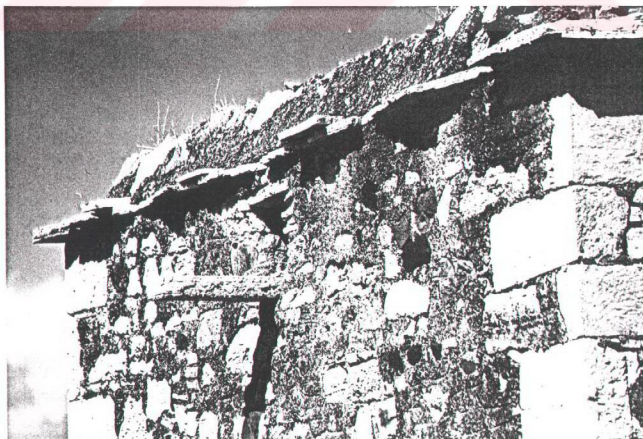
FIGURE.2.118. Flatstone Eave, Rain Gutter
