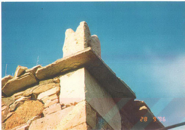
FIGURE.2.145. Decorative Roof Corners, Flatstone Eave
