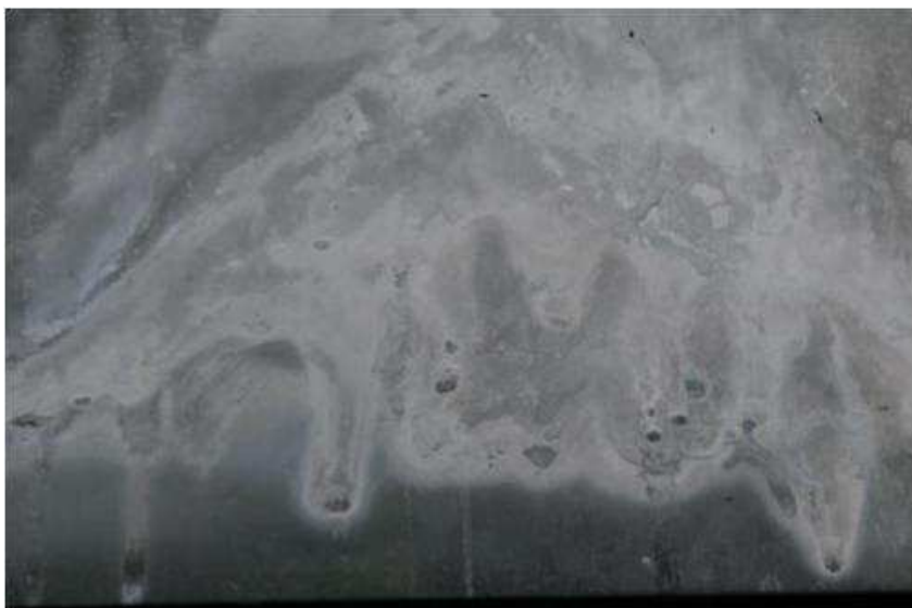
Figure 2.9: A photograph of window glass after long term corrosion by water.
