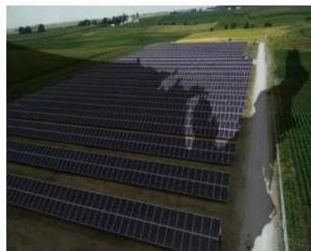
Figure 2.16. Shaded PV system [79].
