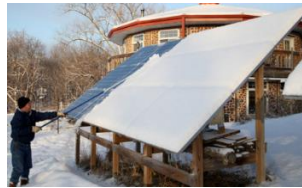
Figure 2.17. PV system is covered with snow.
