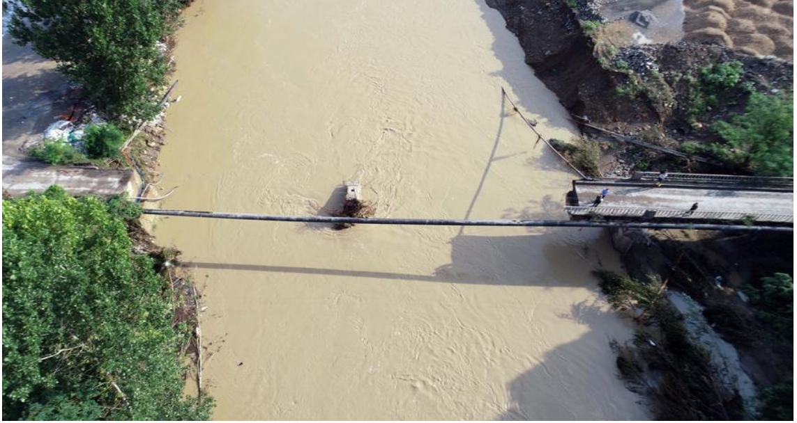
Figure 1.2: Failure of Cevizdere Bridge in Ordu due to flood event
