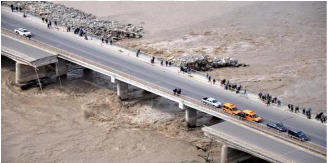
Figure 1.3: Failure of Çaycuma Bridge in Zonguldak due to scour
