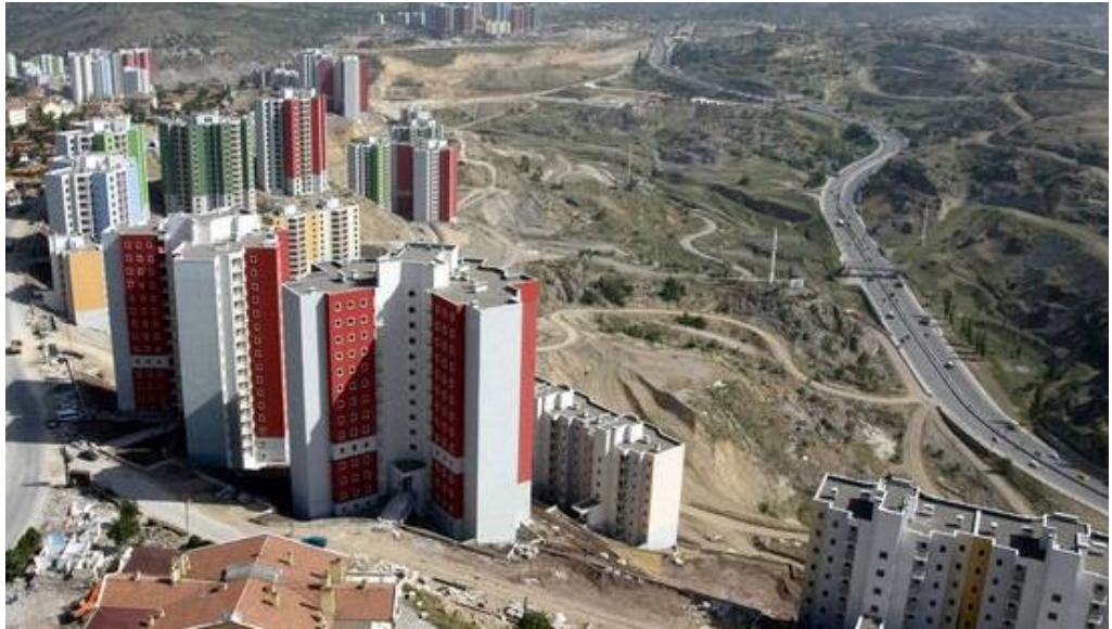
Fig 3.21 Transformation project that was realized by Mass Housing Administration (TOKİ) in the Northern section of Ankara
