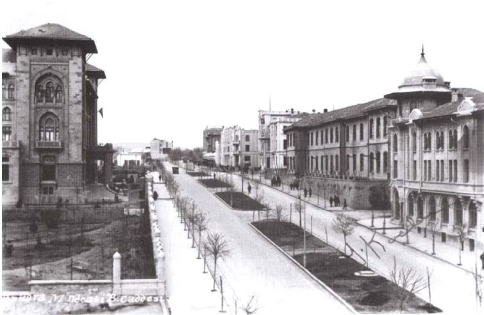
Fig 3.11 Bankalar Street on 1920s: Tekel Başmüdürlüğü (Mongeri) on the right and Ziraat Bankası (Mongeri) building on the left side can be seen
