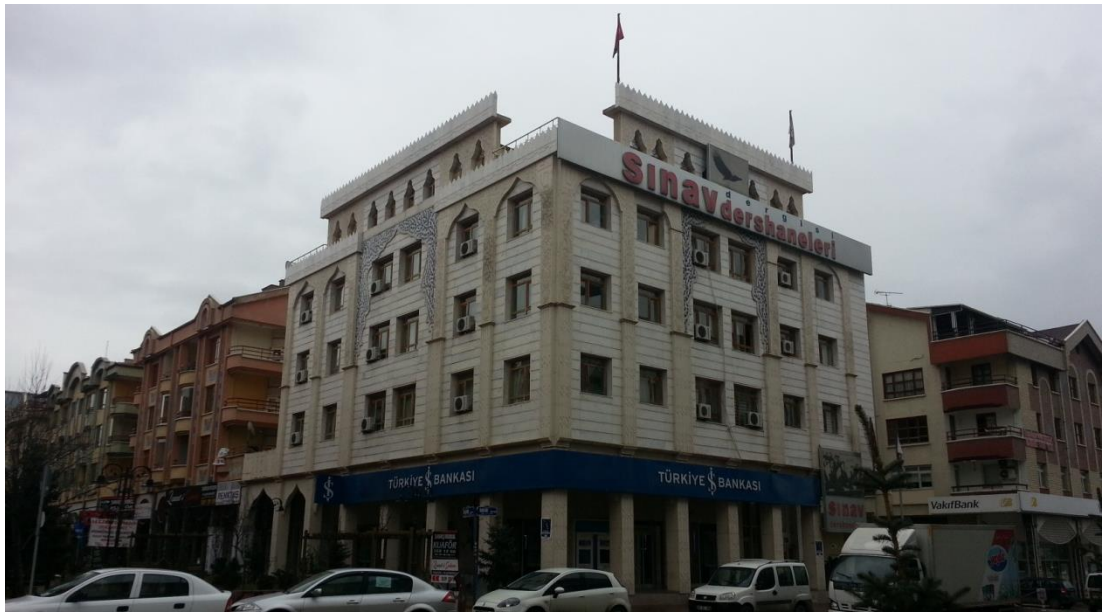
Fig 4.29 General view from Residential Area B
