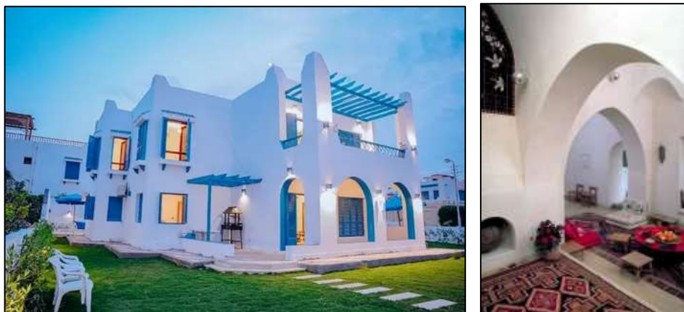
Figure 2.14: Exterior & Interior of a Modern House in Tunis Village Fayoum (Alilatif, 2024).
