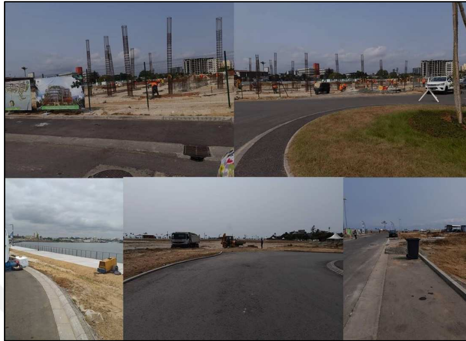
Figure 4.5. The northern area of the project is under construction. The pictures were taken on August 20, 2022, during the opening day of the north promenade
