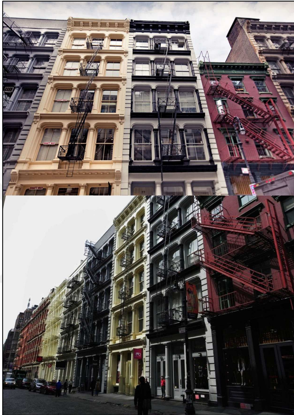
Figure 2.4. Cast iron buildings in SoHo [79]
