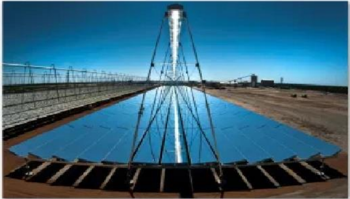
Figure 2.8 Linear Fresnel reflector system “Concentrated Solar Power” (Anonymous,2015).
