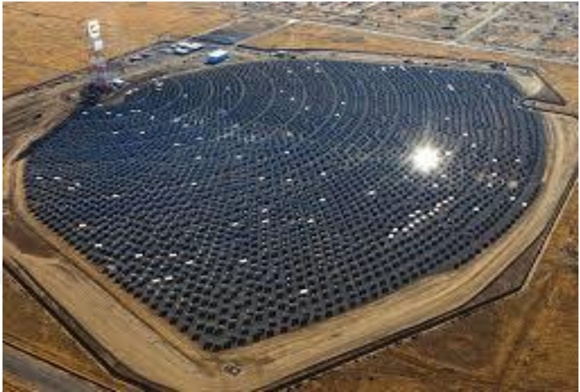
Figure 2.5 Solar tower or central receiver system: Coalinga California (Brightsource, 2011)
