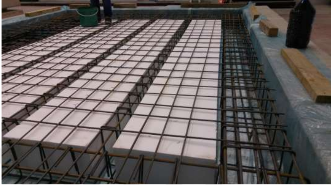
Figure 8. General view of the slab before application of concrete (by Erdemli)
