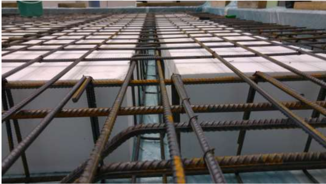
Figure 9. General view of iron reinforcement of girders and EPS block fillers (by Erdemli)
