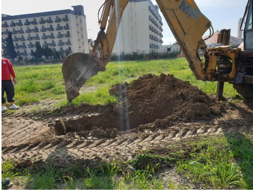
Figure 3.1: The extraction of expansive soil from selected location in South Campus (35°08'51.2" N, 33°54'14.0" E).
