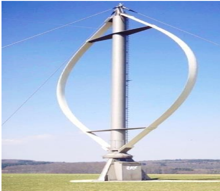
Figure 4.2. Vertical Axis Wind Turbine (Aboufaires, 2015)
