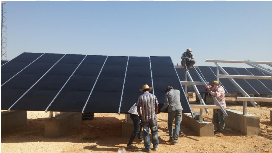
Figure 3. 7 The installation of modules
