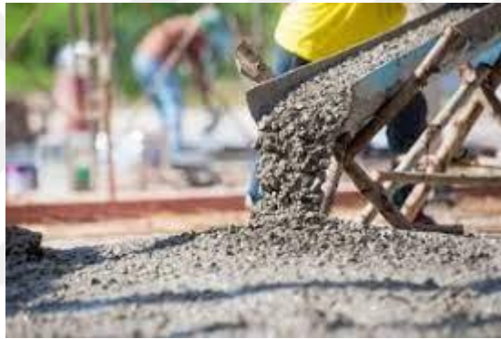
Figure 2.2: High Strength Concrete Production.
