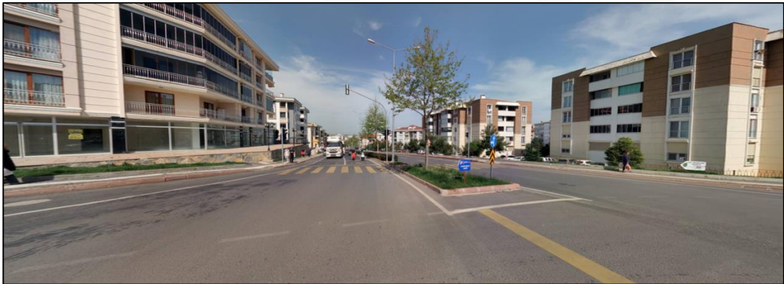
Figure 4.17. Çandarlızade İbrahim Paşa avenue street view from north, photographed by author.
