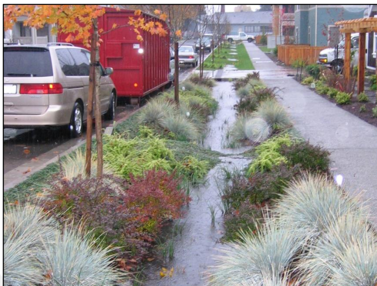
Figure 5.51. Example of a roadside structured rain garden [114].
