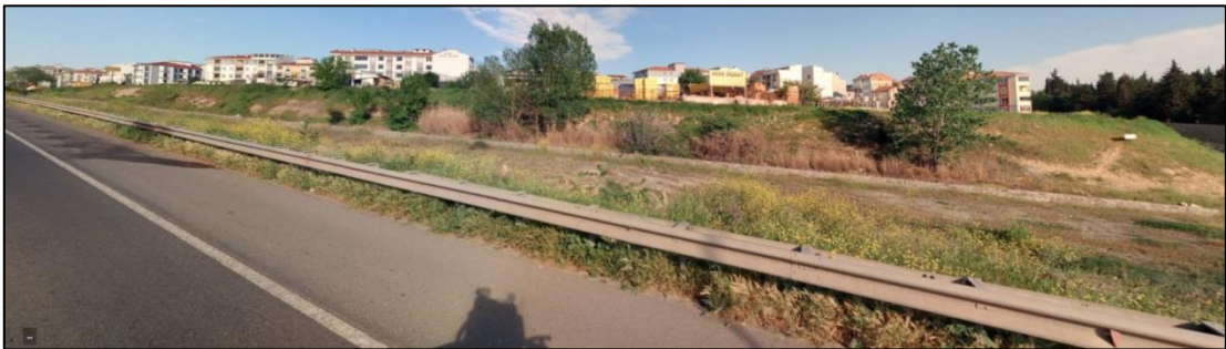
Figure 4.13. Inefficient-use spaces located at the intersection of Kanuni Sultan Süleyman boulevard and Hayrabolu street - 2, photographed by author.
