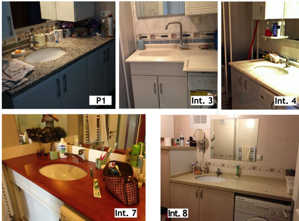
Figure 5.30 : The undercounter washbasins.
