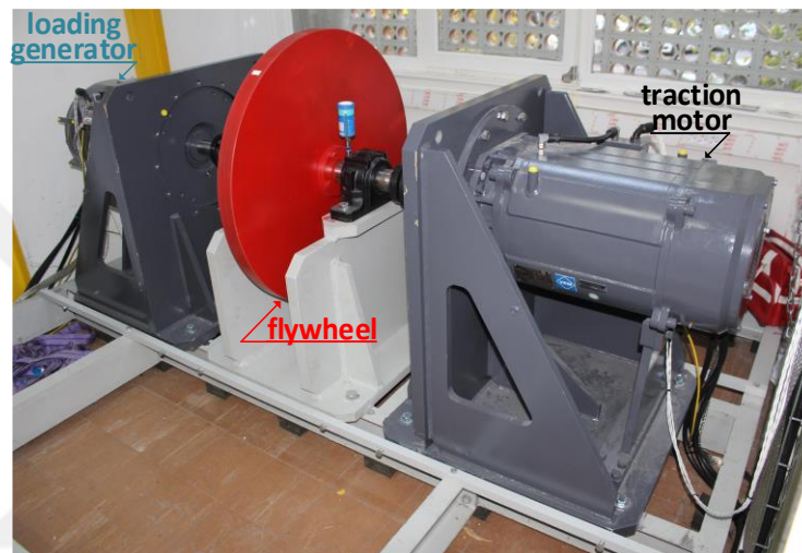
Figure 5.5. Installed motor test bench
