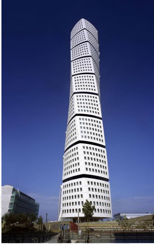
Görsel 3.14 “ Turning Torso ”, Santiago Calatrava , 2005
