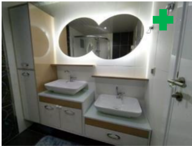
Figure 7a. The sinks with two heights (photo by the author)
